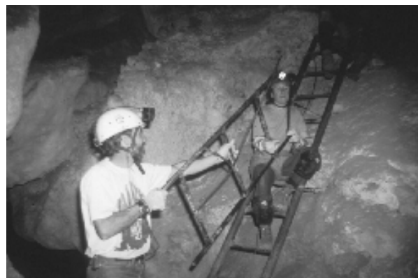
Figure 3. Deemed to be a safety hazard and unnecessary, the metal ladder and a number of other metal structures leading into the New Mexico Room were removed by volunteers from the Pajarito Grotto. (Photo David Jagnow)
